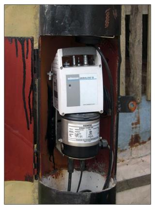
Sebalog Dx data logger connected to a flow meter
