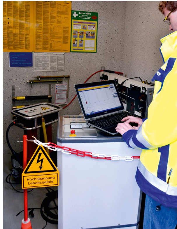
TDS 40 together with the PD detector PDS 60 in operation to test the quality of workmanship on a newly installed cable.
