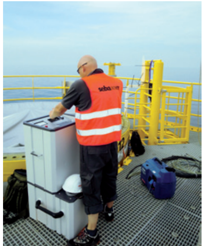
VLF CR-60 kV in operation on the "Baltic 1" wind park (Baltic Sea)
